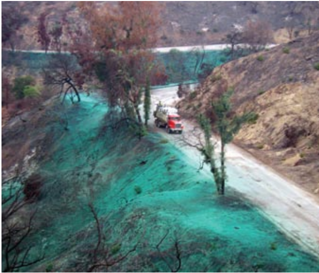
Griffith Park fire project: hydromulching from a ground unit
