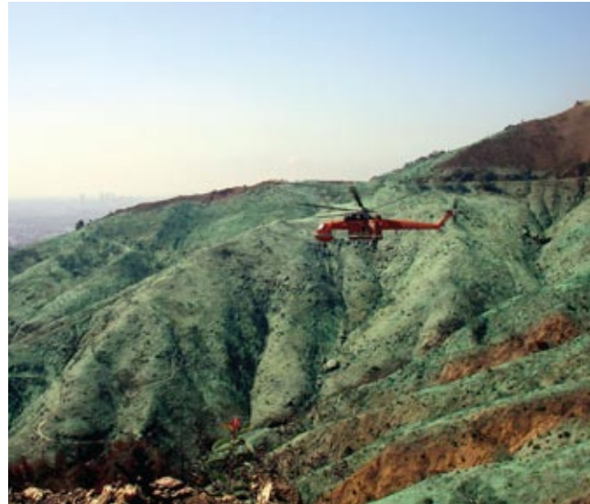
Griffith Park fire project: aerial application of hydromulch via Erickson Air-Crane
